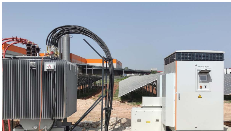
SG3125HV-30 has Max. PV input current up to 3997 Amperes. Max. Efficiency: %99 / European Efficiency: %98.7
